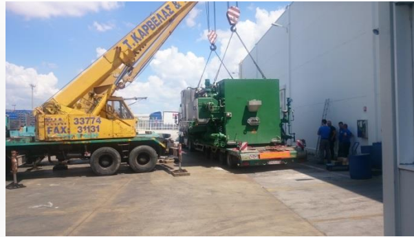
Cranes are set to unload
